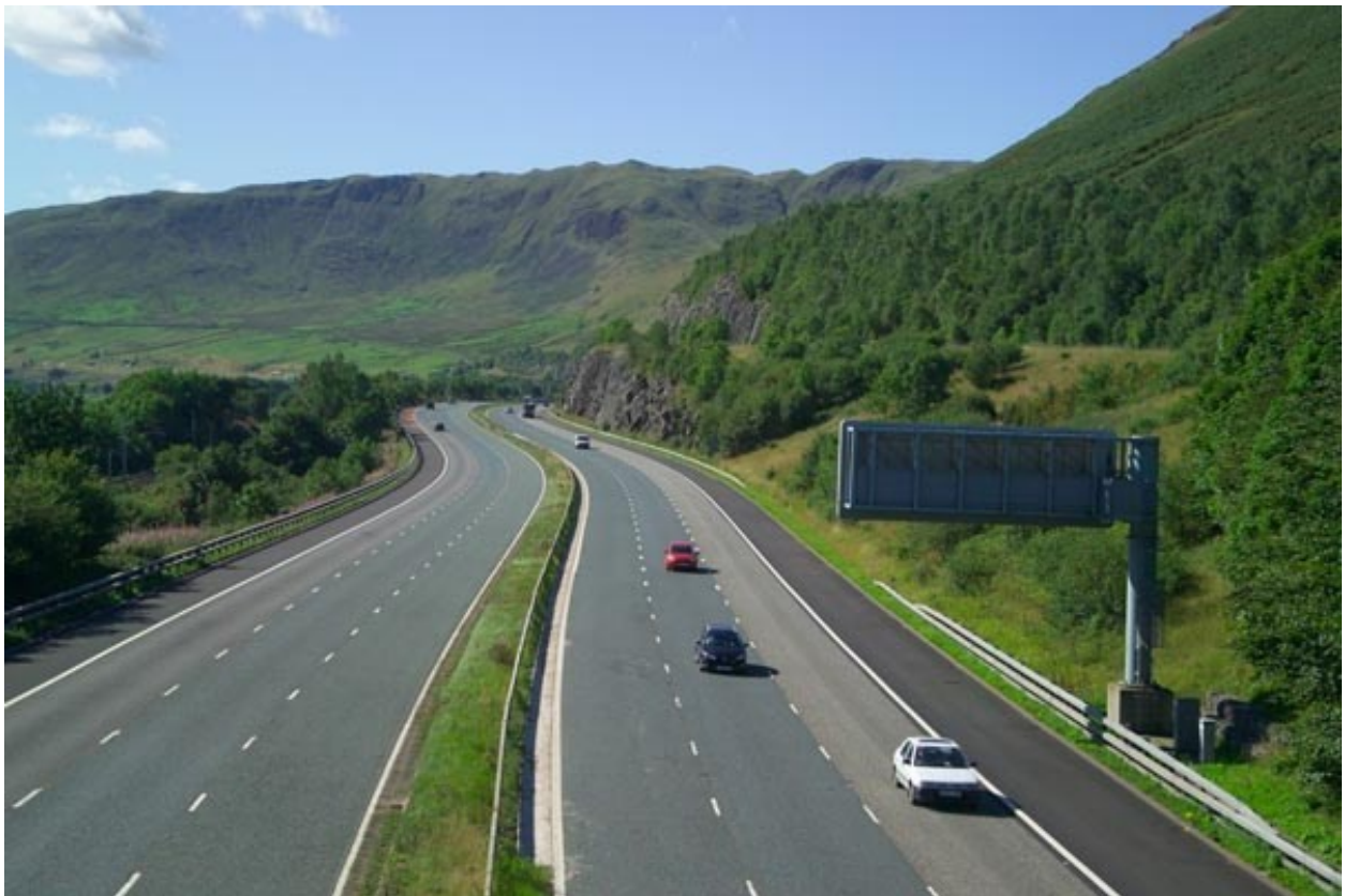
Islamabad – Peshawar Motorway
